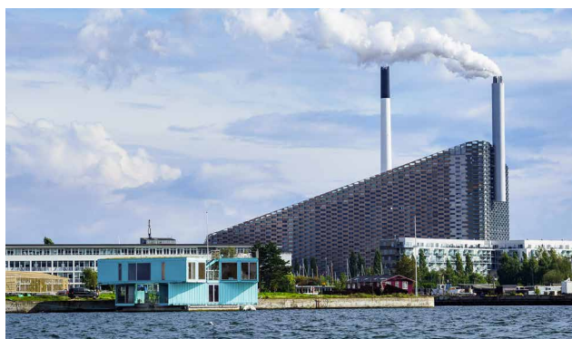
The waste incineration plant Copenhill also serves as an activity centre
